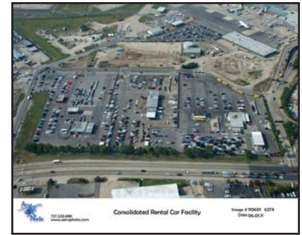
Consolidated Rental Car Facility
