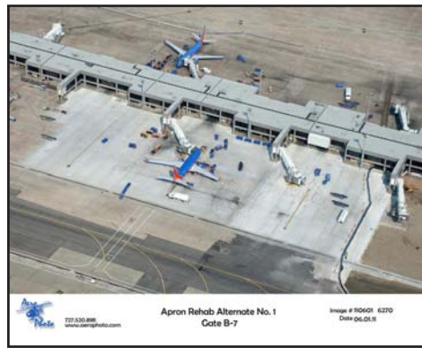
Apron Rehabilitation - Concourse B
