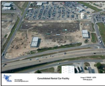
Consolidated Rental Car Facility
