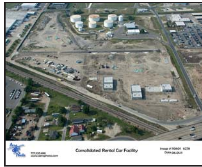
Consolidated Rental Car Facility
